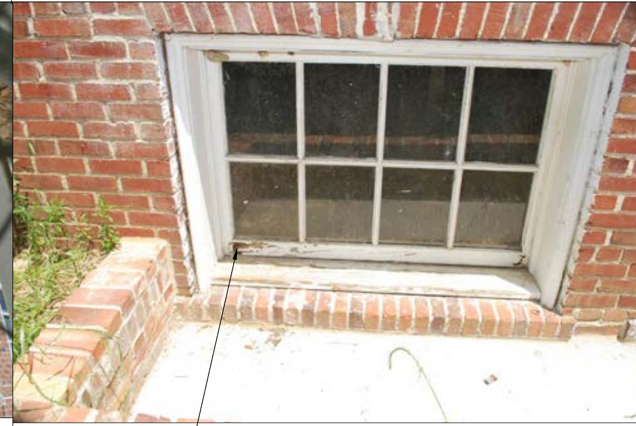
3 EAST ELEVATION WINDOW SILL REPAIR
