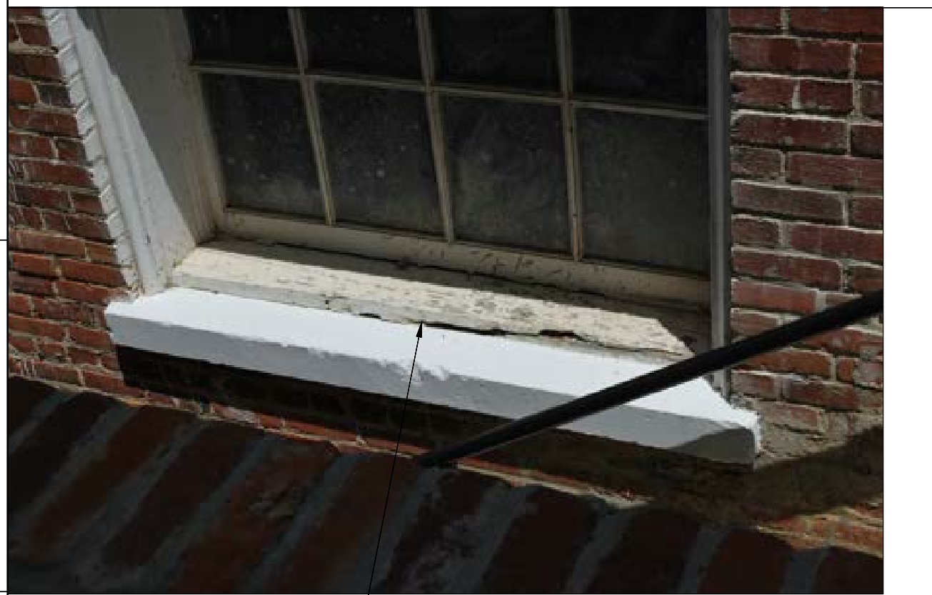
4 EAST ELEVATION WINDOW SILL REPAIR
