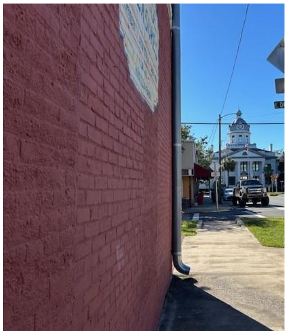
BRICK SURFACE DETAIL
